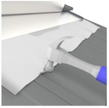
Using a hammer or rubber mallet, gently form the Soft Flash to the tile profile.
